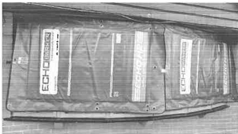
Figure 6: EchoBarrier window coverings in place
